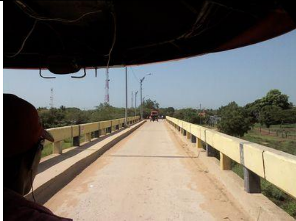
Long bridge outside of Pivijay
